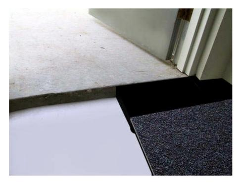
Picture 12-4 Recessed Sub-floor at Door Opening with full carpet tile overlaying perimeter and sub-floor seam
