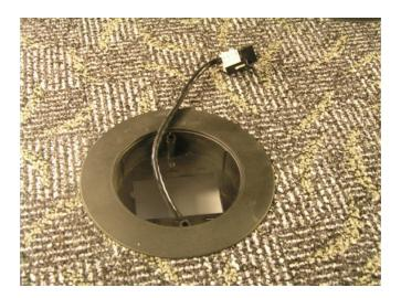
**Connector snaps into Mounting Plate**
