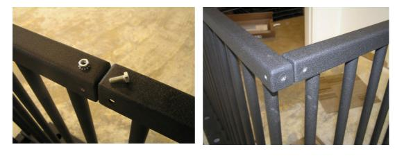
Bolt is placed through the appropriate holes of the rail top cap, from the underside, and tightened.
