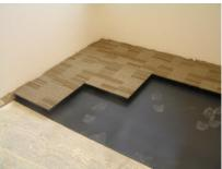
When starting the System at a corner with an obstacle, use three whole panels to determine the area around the obstacle. Corner area needs to be filled with appropriate perimeter / pedestal components and cut in around the obstacle, to provide a firm starting point.
