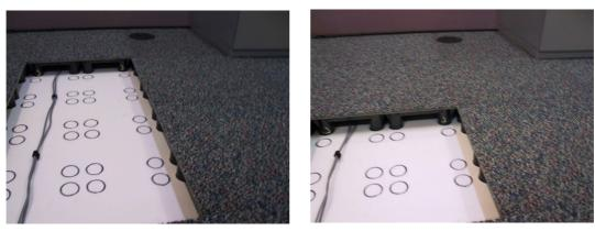
If your relocation requires more cable length than is available, disconnecting the existing cable and reconnecting a new cable from the outlet is required.
