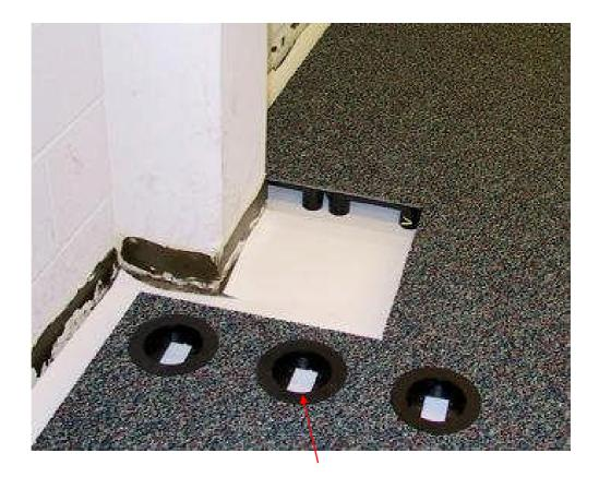
An appropriate quantity of whole panels will be supplied with outlet ports installed into them, per the project drawing. These outlet locations are provided with a universal outlet grommet (Powerport grommet) which is used for the installation of either electrical or communication components.
