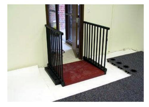
Rails configured at angles to provide ADA Wheelchair Turnaround
