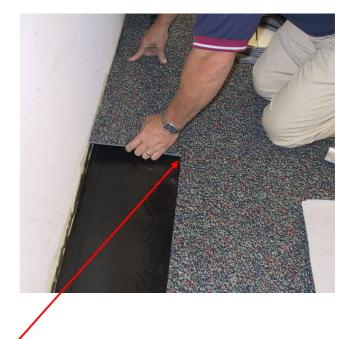
Please Note !!! All cut carpet tiles should be placed so that the factory edges (not cut edges) adjoin the factory edges of adjoining tiles. Cut edges are always placed against walls, rail bases, Z Trim, etc.)
