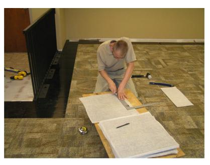
Picture 8-11 Carpet Tile seam installed beyond top and bottom of ramp
